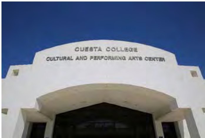
BUILDING IDENTIFICATION SIGNAGE
