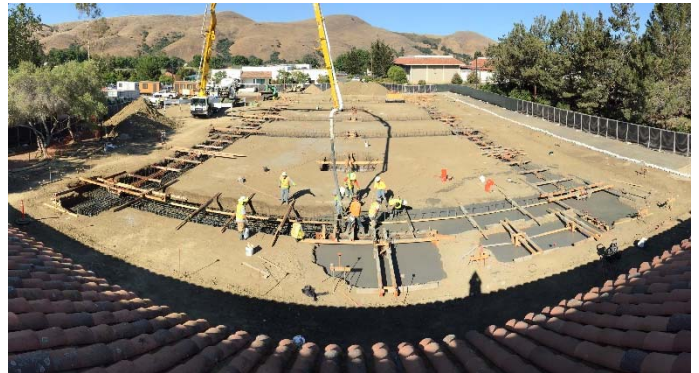
ABOVE: Concrete foundations being placed for the SLO Instructional building.
