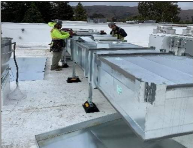
ABOVE: New ductwork being installed
