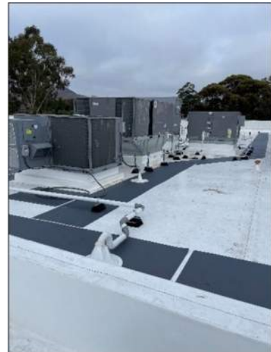
ABOVE: New single-ply roofing and HVAC
