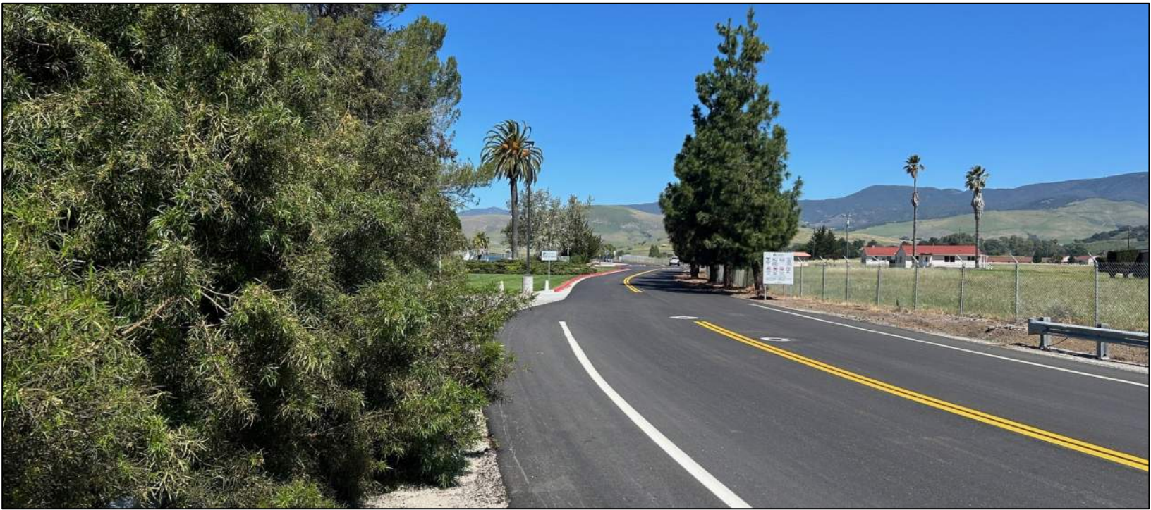
ABOVE: Asphalt Replacement Project.
